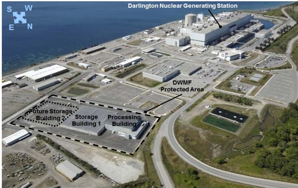
Figure 2: OPG's Darlington Waste Management Facility (Source: OPG)
